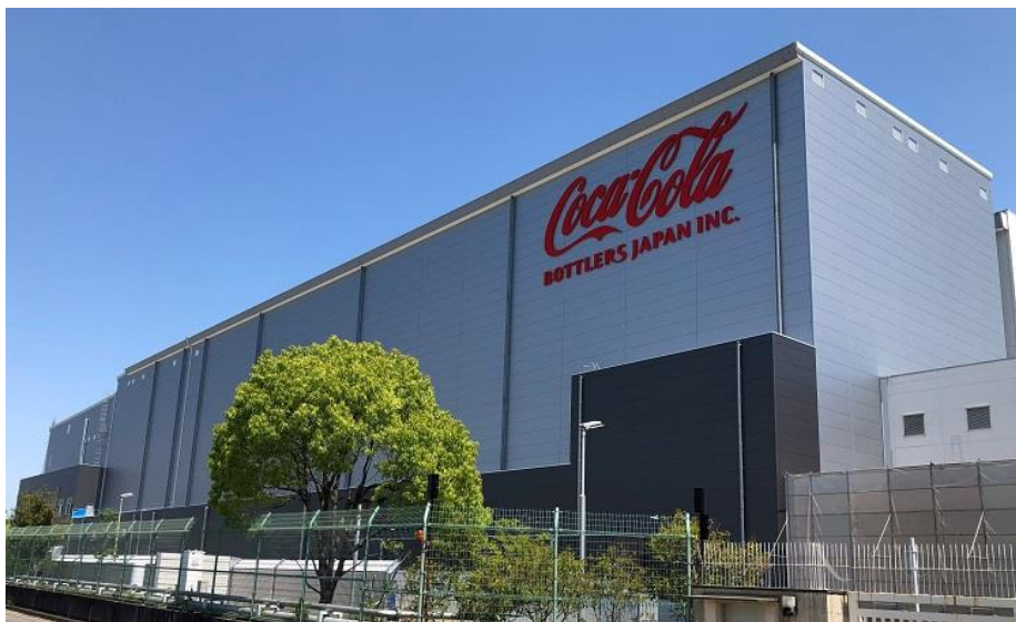
Exterior view of the Akashi Mega DC
