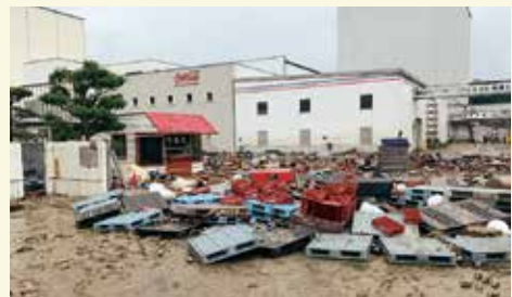
Hongo Plant after the flooding
